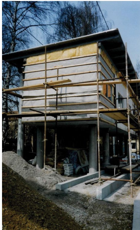
Gradnja dveh dodatnih kabin za radio in televizijo Construction of two additional cabins for radio and television 2001
